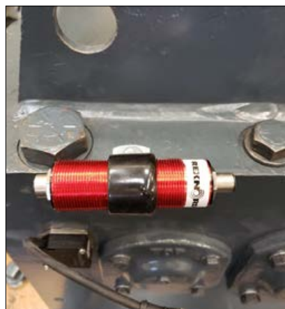
Figure 7 – Converter Installed on A+Plus Drive on top ledge
