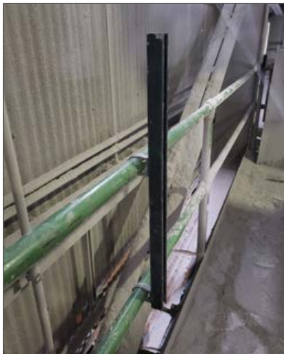
Figure 15 – Remote installation of Unistrut on rail
