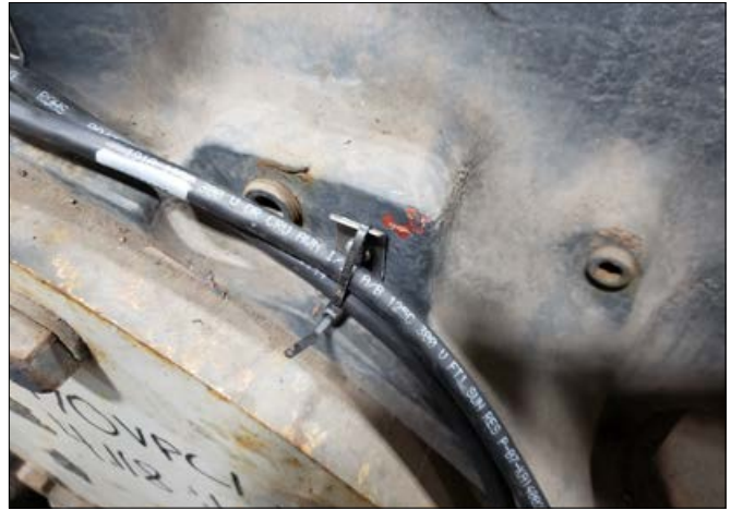
Figure 24 – Sensor cables secured with cable tie mounts
